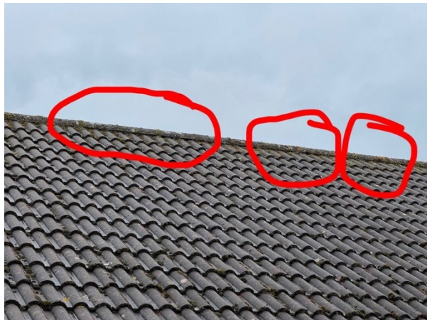
Picture 4 – Strip loose ridges on main roof. Clean all old cement off ridges & Replace with dry ridge system.
