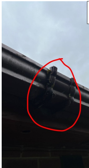
Picture 6 – Replace any broken joiners and gutter clips.
