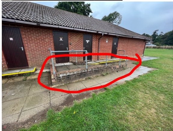
Picture 3 – Replace missing bricks, remove broken bricks and re cement.
